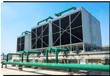
Figure 3) Cooling Towers on a Roof
